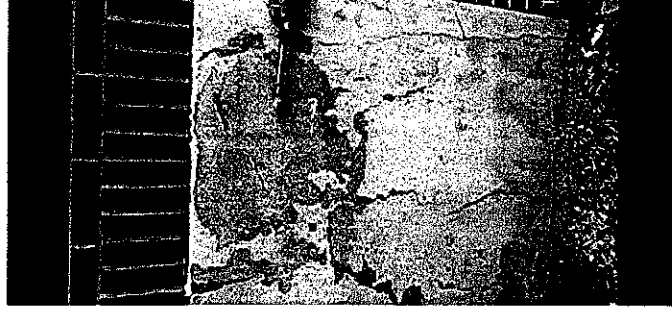
(Delaminated Concrete)
